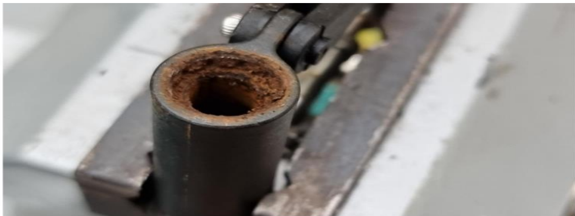
Main Boom Arm Bearings Rusted out – Outer Race Casing still to be removed before New bearing can be fitted
