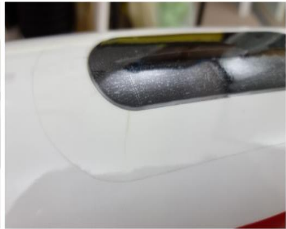
Application of Clear Mylar Tape to seal water leaks
